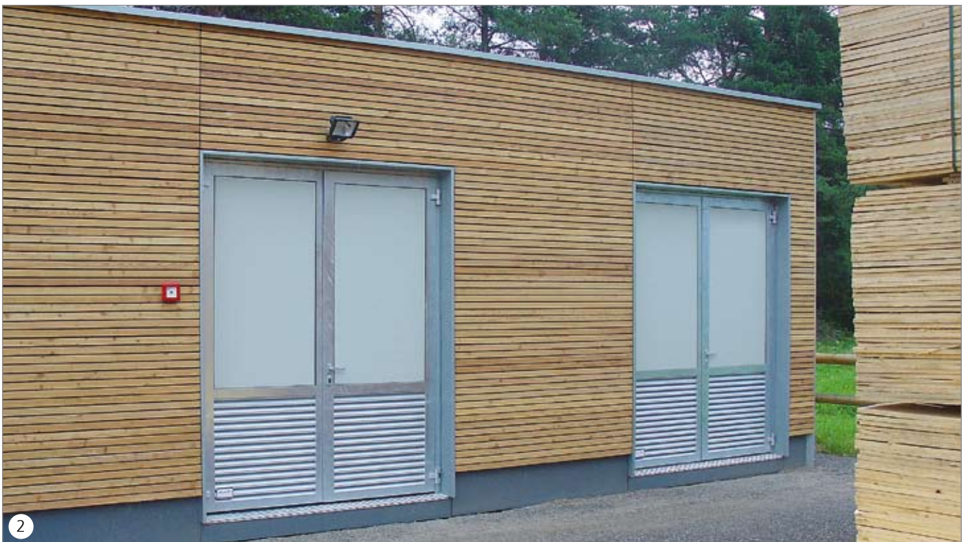
Doppelflügeltür belüftet - Stahlschalung ventilated double leaf door – lateral steel coating
