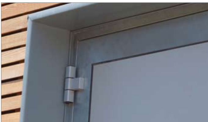
Stahlschalung der Doppelflügeltür in der Fassade lateral steel coating of the double leaf door in the facade
