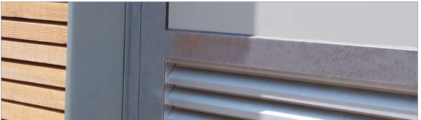
Stahlschalung der Doppelflügeltür in der Fassade lateral steel coating of the double leaf door in the facade
